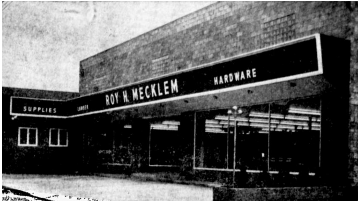
The Roy H. Mecklem lumber and hardware store in Monaca, Pennsylvania, at the time of the grand opening in 1954
